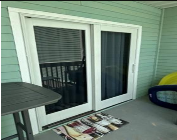
Photo 19 View of balcony sliding glass door in good condition.
