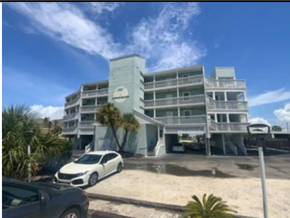
Photo 1 Overall view of north elevation.
