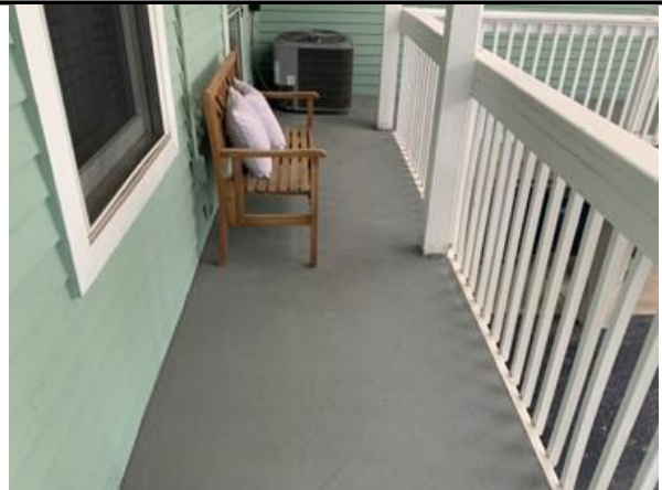
Photo 4 View of common walkway.
