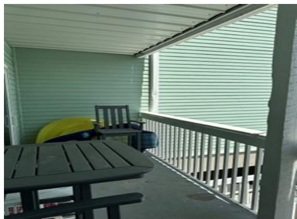
Photo 18 View of balcony decking in good condition.
