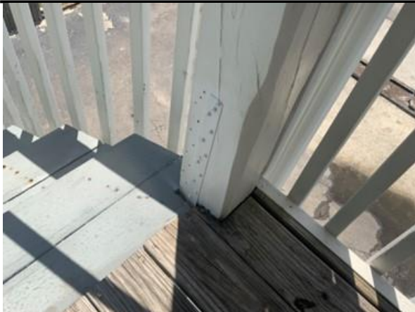
Photo 7 View of hurricane straps in good condition.
