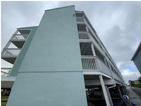
Photo 2 Overall view of stucco cladding.
