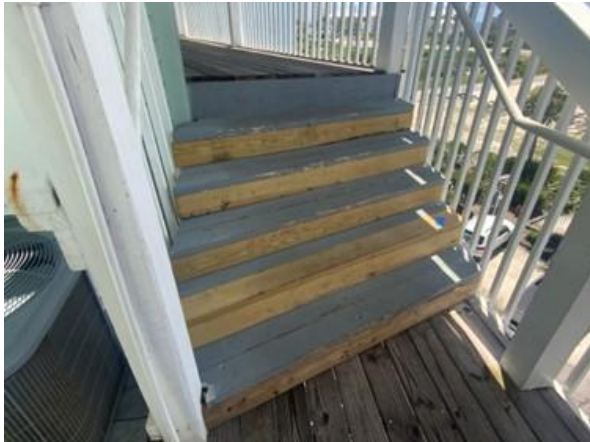
Photo 8 View of wood stairs in good condition.
