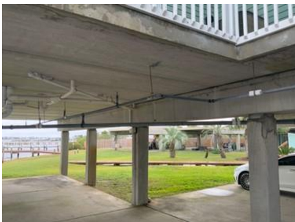
Photo 3 Overall view of concrete columns in good condition.
