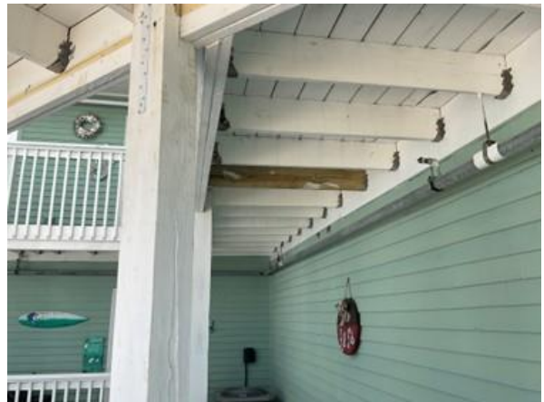
Photo 17 View of vinyl siding in overall good condition.
