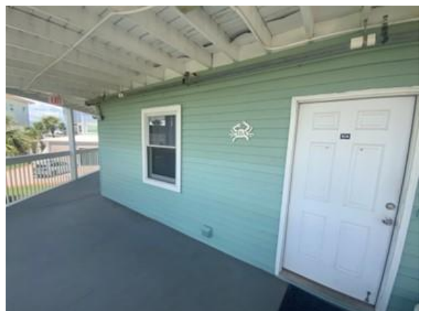
Photo 6 View of unit entry doors and windows in good condition.
