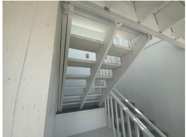
Photo 11 View of wood stairs in good condition.
