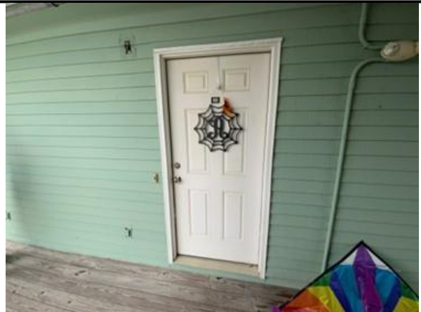
Photo 16 View of unit entry door in overall good condition.
