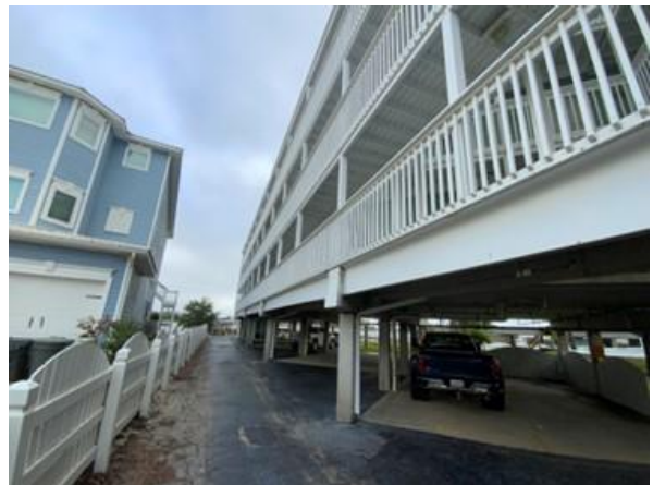
Photo 12 Overall view of west elevation of building.
