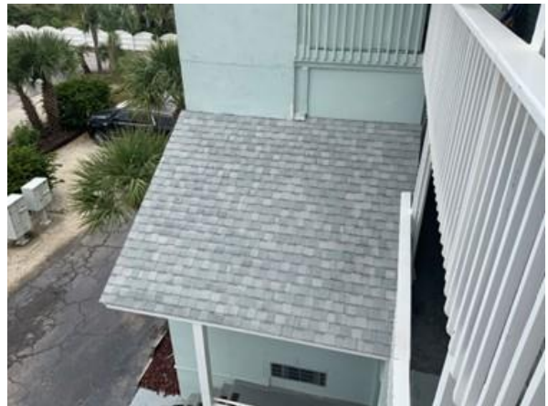
Photo 5 View of roof in good condition.
