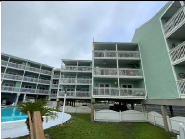
Photo 13 Overall view of north elevation.
