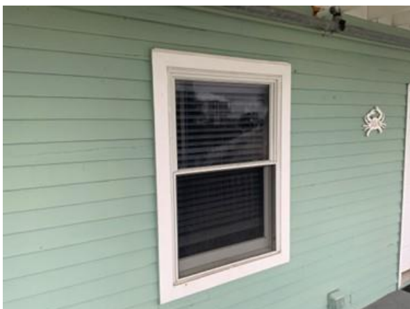
Photo 15 View of exterior window in overall good condition.
