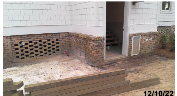
Stair Side Entry
