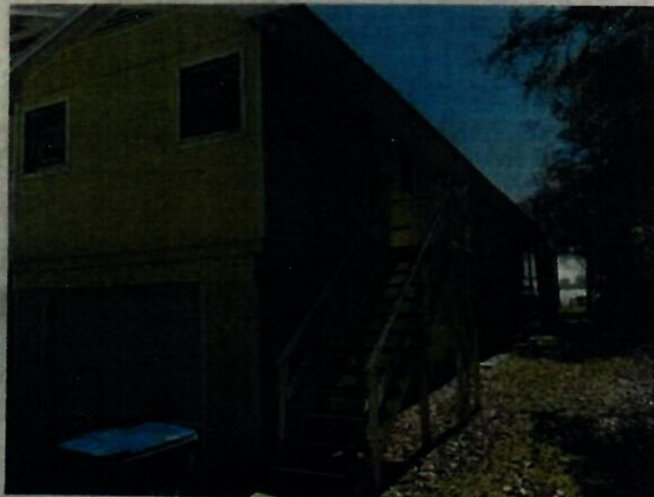
WEST SIDE VIEW 12/21/17
