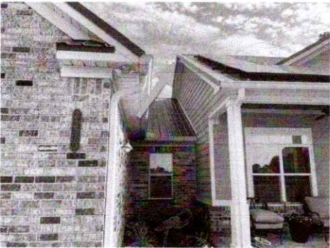
Fascia board covering missing
